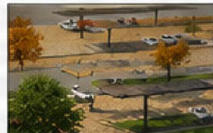
PARKING WITH SOLAR CANOPY
